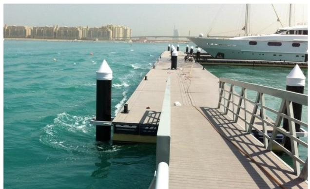
Pontoons acting as wave breakers at Mina Seyahi
