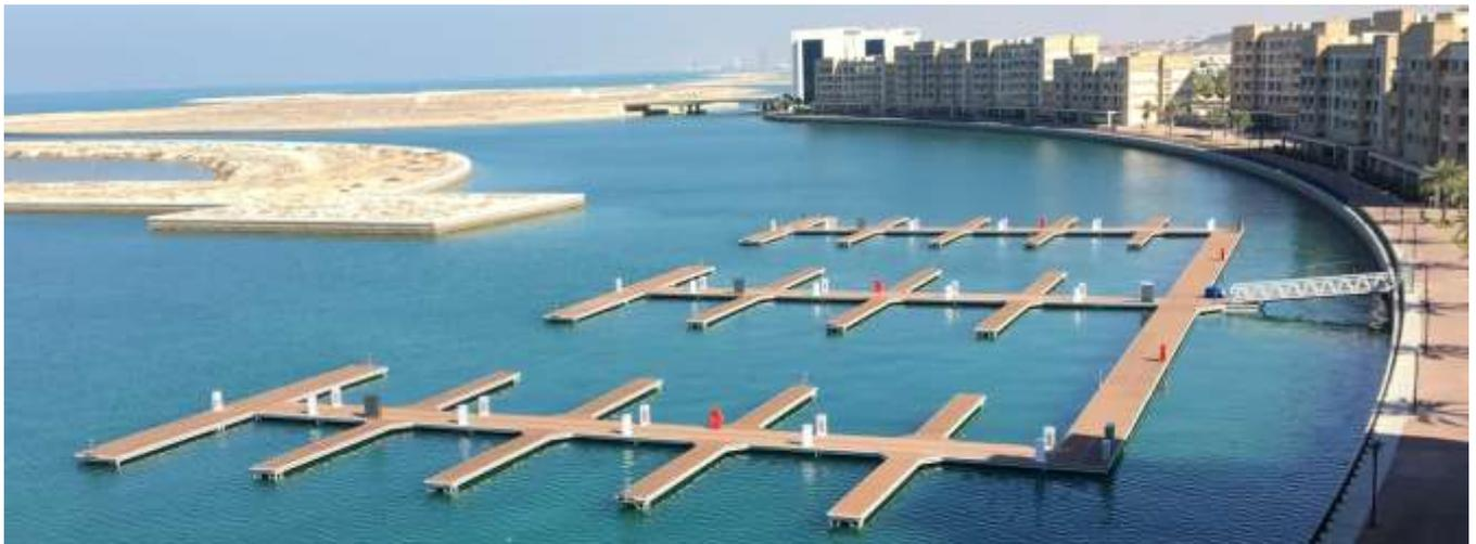
Photo of frame and float fibre reinforced polymer pontoons installed at Taweela Port Marina, Abu Dhabi, United Arab Emirates for Command of Military Works and Marfa Fisherman's Port, Abu Dhabi, United Arab Emirates for Abu Dhabi Ports Company
